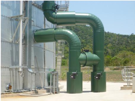
surface having dry bulb temperature (DBT) lower than the dew point temperature (DPT) of the air in contact with that surface. DPT is conditional on the relative humidity (RH) and DBT of the air around the pipe.
